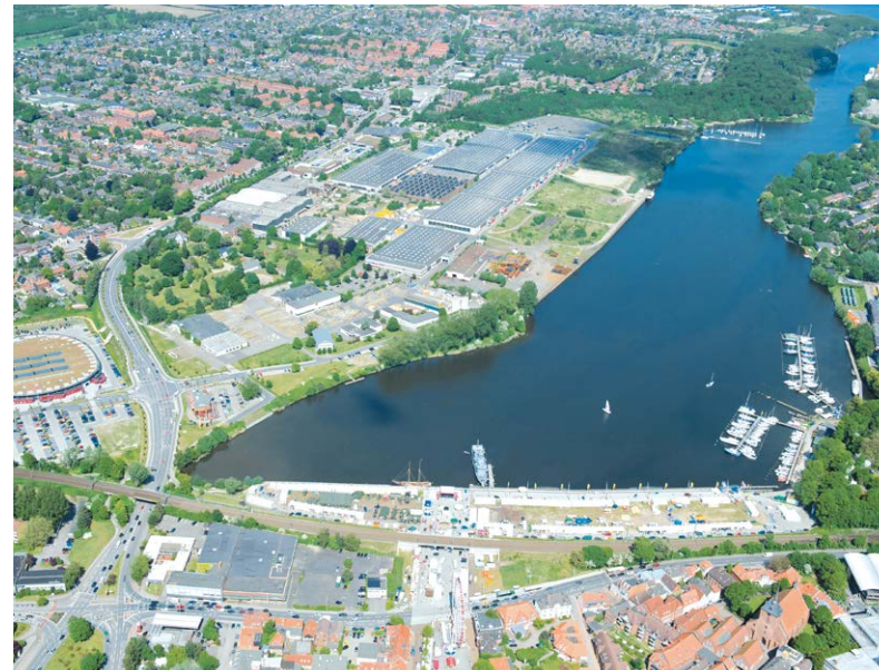
Headquarters of the ACO Group in Rendsburg/Büdelsdorf
